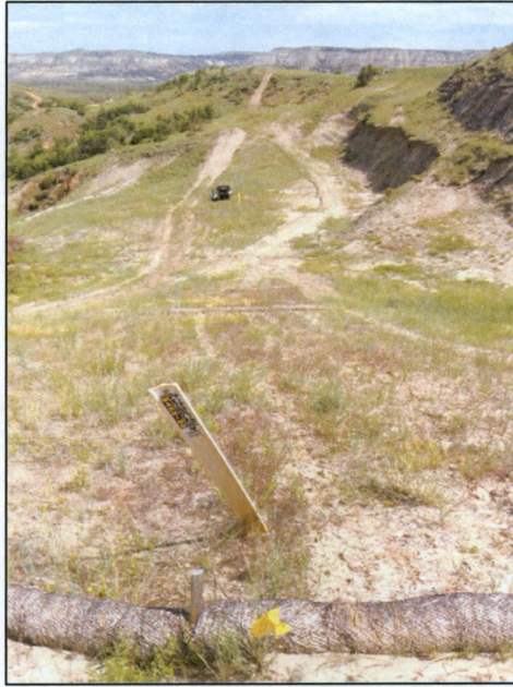
Photograph 1. Vantage of regraded fill area along existing Bridger Four Bears pipeline. View to north.
